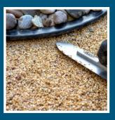
4. Compact the stones using a trowel, or by standing on wooden planks. A flat surface will be a lot more robust than with protruding stones when subjected to foot traffic.
